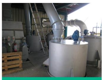
Figure 2: Inert feeding system.
